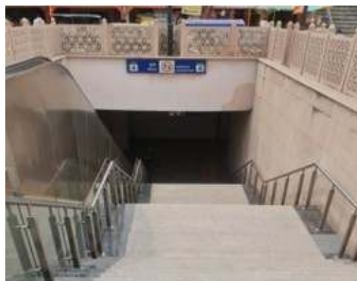
Station Entry to Concourse Level
